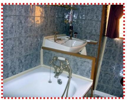
This is a diagram of the under sink area. I first had to pencil shape for the cut out area. I then stuck the tiles and when fully dried, I cut out the shape with a tile saw.
